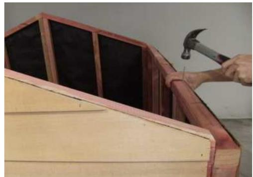
Step 10: Using 30mm clouts nail top cedar boards to Stiffeners (2-3 per board). Pre-drill holes to stop boards from splitting.
