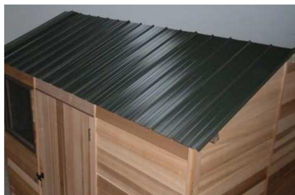
Ensure purlins are straight, nail roof sheets to purlins, 1 nail per pan.
