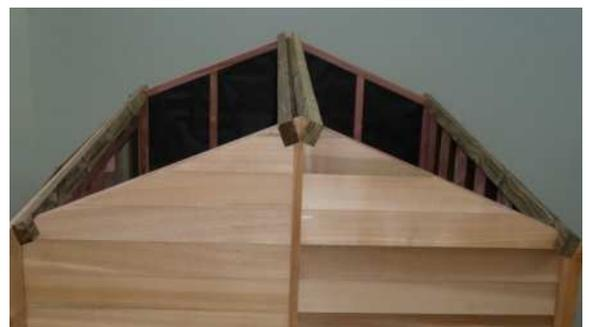
Step 14: Using 1 x 75mm tek screw, screw bottom purlin to top plate centrally in shed.
