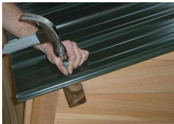
Step 17: Lay out remaining full roof sheets and 1/2 sheet. Rivet these sheets together, 2 rivets per joint, to make 1 large roof panel as shown in photo. Tack remaining top corner and bottom corner ensuring edge of sheet is flush with end of purlins and height is correct.
