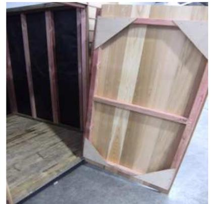
Step 21: Using 3 x 75mm tek screws, screw door stud to panel ensuring height is correct.
