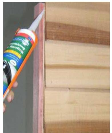
Step 7: Silicone and nail remaining beads on each panel. Screw panels together using 3 tek Screws per join and 4 on the longer joins on gable end panels.
