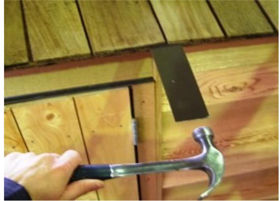
Step 22: Nail using 50mm nails, above the bottom of the next row of shingles.
