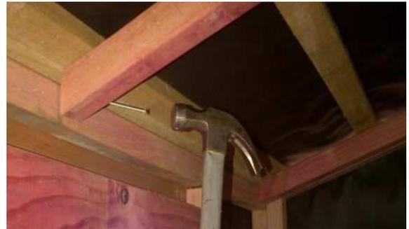
Step 18: Using 6 x 75mm tek screws , screw 3x collar ties to underside of rafters. Pre-drill before screwing if necessary.
