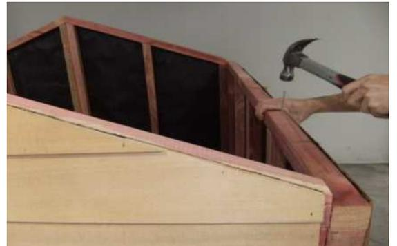
Step 10: Using 30mm clouts nail top cedar boards to stiffeners (2-3 per board). Pre-drill holes to stop boards from splitting.
