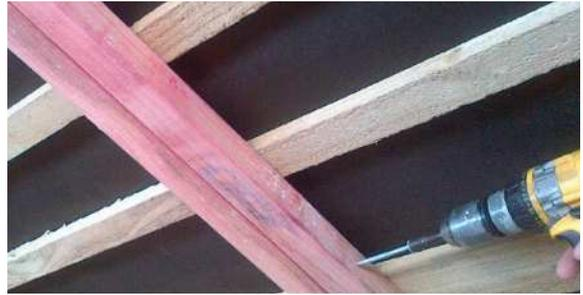
Step 17: Using 12 x 75mm framing nails, nail roof rafters to front and back top plate stiffeners. Pre-drill if necessary.
