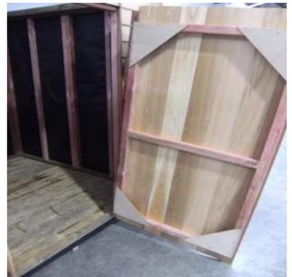
Step 27: Using 3 x 75mm tek screws, screw door stud to panel ensuring height is correct.
