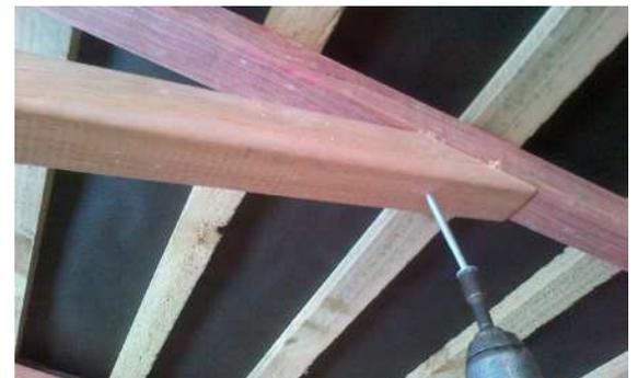
Step 19: Attach a plywood gusset to each side of rafters as shown using 8 x 30mm clouts per side.
