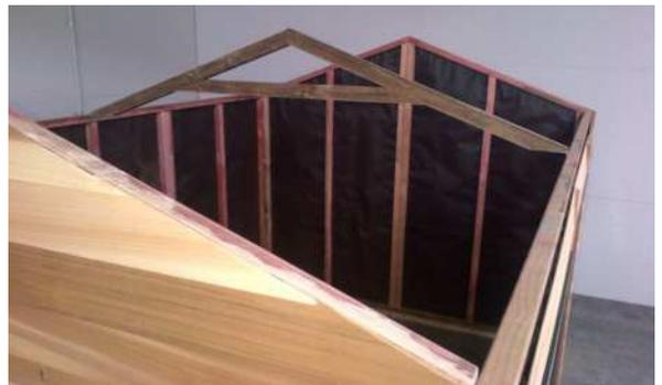
Step 14: Position 8 purlins on roof. Top purlins should be together and bottom purlins should be against top plate. Using 75mm framing nails, predrill then nail purlins into top of gable end panels and truss (2 nails per join).
