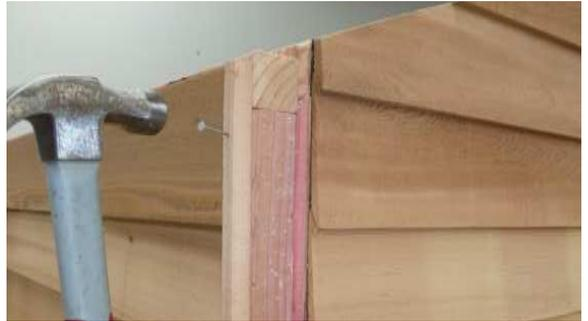
Step 12: Silicone and nail corner clashing on all corners as shown using 5 x beading nails per clashing.
