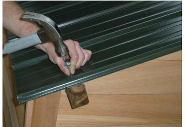
Step 17: Lay out remaining full roof sheets. Rivet these sheets together, 2 rivets per join, to make 1 large roof panel as shown in photo. Tack remaining top corner and bottom corner ensuring edge of sheet is flush with end of purlins and height is correct.
