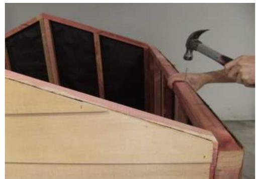
Step 10: Using 30mm clouts nail top cedar boards to stiffeners (2-3 nails per board). Pre-drill holes to stop boards from splitting.
