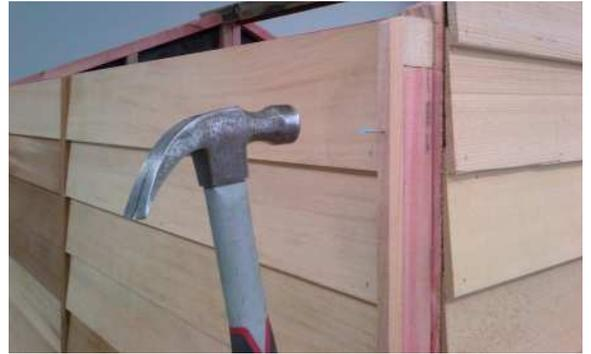
Step 12: Silicone and nail corner clashings on all corners as shown using 5 x bead nails per clashing.
