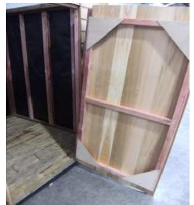
Step 21: Using 3 x 75mm tek screws, screw door stud to panel ensuring height is correct.
