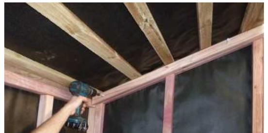
Step 15: Using 2 x 75mm framing nails, nail centre rafter to front and back top plate stiffeners. Pre-drill if necessary.
