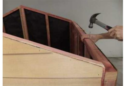
Step 9: Using 30mm clouts nail top cedar boards to stiffeners (2-3 per board). Pre-drill holes to stop boards from splitting.
