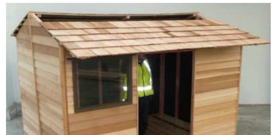
Step 14: Using 75mm tek screws, screw roof panels into end wall panels, (2 screws each end per panel), ensuring end of rafter lines up with centre of gable panel.
