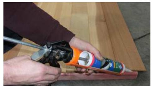
Step 7: Silicone and nail remaining beads on each panel. Screw panels together using 3 tek screws per join and 4 on the longer joins on gable end panels.
