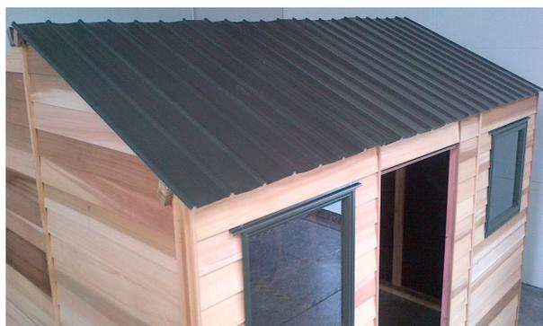
Ensure purlins are straight, Nail through the pan using 30mm clouts into the top purlin, using 50mm roofing screws with washers screw through the rib into the bottom purlin.
