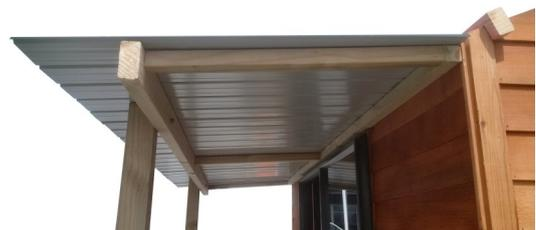
***Continue to nail Cedar shed roof as in step 15. Once shed is finished attach veranda barges and spouting.***
