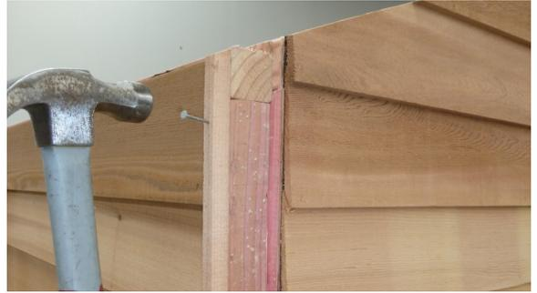
Step 12: Silicone and nail corner clashings on all corners as shown using 5 x beading nails per clashing.
