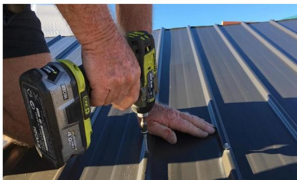
Step 17: Lay out remaining full roof sheets and 1/2 sheet. Rivet these sheets together, 2 rivets per joint, to make 1 large roof panel as shown in photo. Tack remaining top corner and bottom corner ensuring edge of sheet is flush with end of purlins and height is correct.
