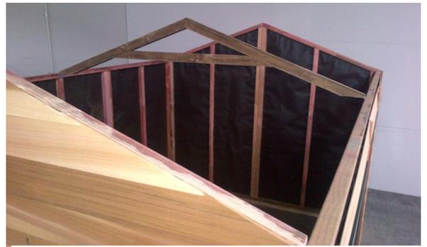
Step 14: Position 12 purlins on roof. Top purlins should be together and bottom purlins should be against top plate. Using 75mm framing nails, predrill then nail purlins into top of gable end panels and truss (2 nails per join).
