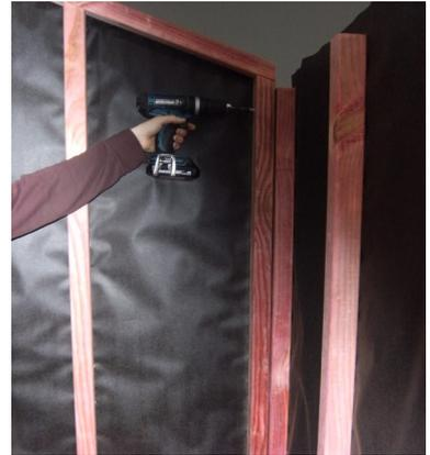
Step 6: Silicone edge of weatherboards on standing panel and nail on cedar beads with 5 x bead nails. (Refer to wall plan for correct beads). Make sure bead is properly sealed to avoid leaks. Note: On standard panels only, top of bead is bevelled to allow for slope of roof.
