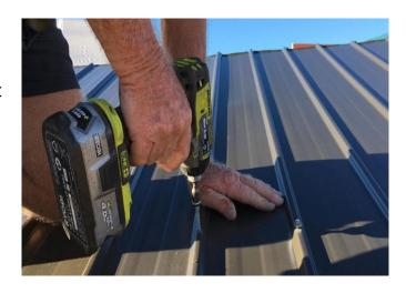
Step 18: Lay out remaining full roof sheets. Rivet these sheets together, 2 rivets per join, to make 1 large roof panel as shown in photo. Tack remaining front corner and back corner ensuring edge of sheet is flush with end of purlins and front overhang is correct.
