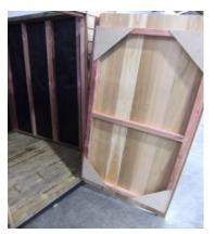
Step 21: Using 3 x 50mm Framing screws, screw door stud to panel ensuring height is correct.
