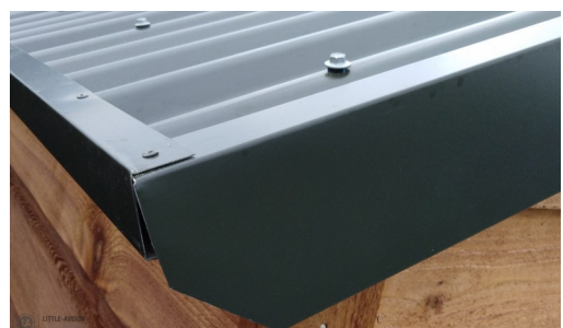
Above shows the ridge flashing, below shows the barge flashings.
