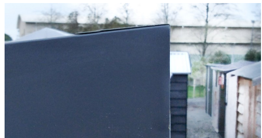
Above shows the ridge flashing, below shows the barge flashings.
