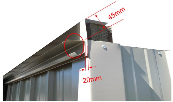
**Step 2:** Hang door in the Door Track. At the right hand end of Door Track, adjust up or down so that the Door hangs parallel with shed. Fit one rivet at right hand end to hold in place. Repeat with left hand end of track.
