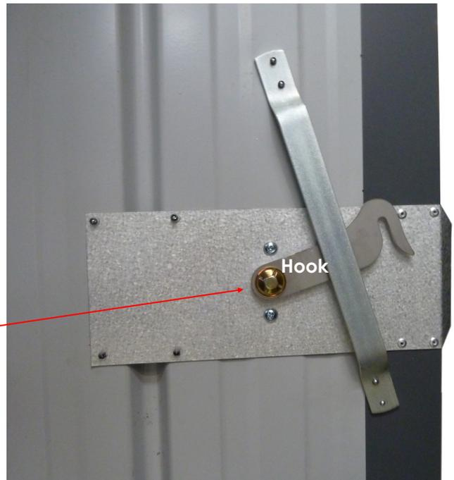
**Step 2:** Once door is hung, position the Locking Stays so they slide into the Locking Brackets easily. Screw Locking Stays to Door Jamb.
