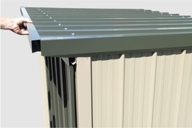
**Step 1:** Position Barge Flashing (G102) on gable ends. Position a Spouting (A103) and rivet to the Barge Flashing at each end. Repeat with other Spouting.
