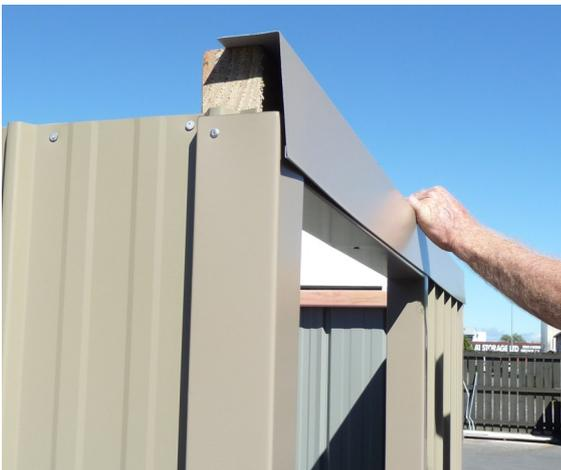
**Step 5:** Position Ridge Cover (A109) on Ridge Beam. While holding straight and square, nail top of Ridge Cover Flashing to Ridge Beam using three 30mm clouts. Rivet front of Ridge Cover to Ribs and Flashings using seven rivets.
