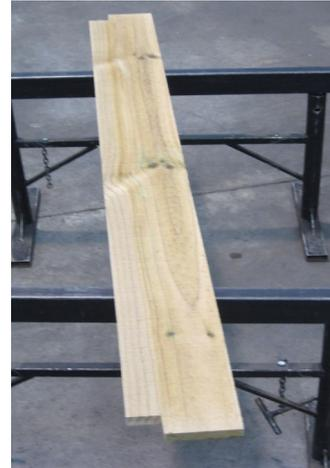
**Step 3:** Re-position Floor Board. Lay out remaining Floor Boards checking around Studs as you go. The last Floor Board may have to be cut to size.
