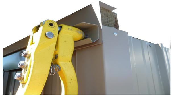
**Step 3:** Remove the Door. Pre-drill and screw another 2 screws between centre screw and the rivets at each end (5 screws per track). Screw track using 45mm door track screws.
