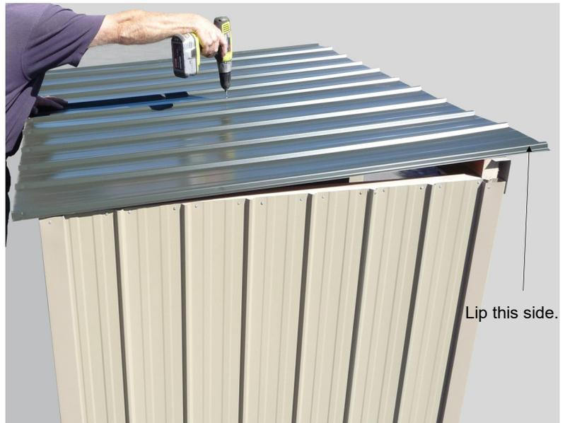
**Step 3:** Position roof so that the front overhang measures 140mm. Line up Ribs on the Roof Sheets with Ribs on the Wall Sheets. Ensure plates are straight then screw roof to Top plates using one 50mm Roofing Screw on each Rib front and back.
