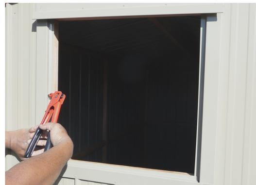
**Step 6:** From the outside of the shed, place glass in Window Frame. Attach a Glazing Bead (G100) with three rivets to each side of the Window Frame to hold glass in place. Pre-drilling Glazing Beads is recommended.
