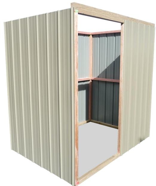
**Step 4: Nailing Off:** Nail one 30mm Clout each side of the Rib (two per Pan) into the Top Plates and Bottom Plates. Nail Wall Sheets to mid wall Nogs (one per pan). Nail each corner Wall Sheet to Studs using two 30mm Clouts evenly spaced.
