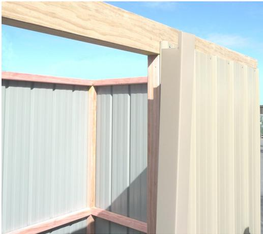
**Step1:** Fit Door Jamb Flashing (104) in between Top and Bottom Plates and hard against Stud. Attach Door Jamb Flashing with three rivets into Rib on the outside and three 30mm clouts into studs on the inside. Repeat with the other Door Jamb.
