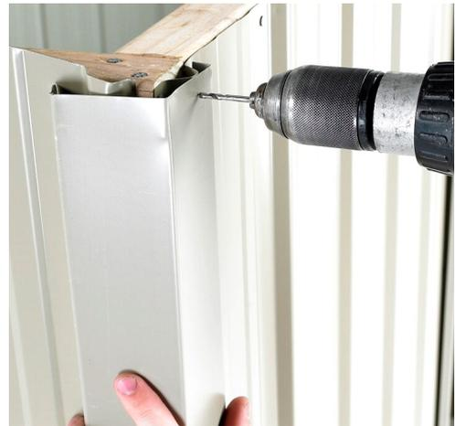
**Step 4:** Fit remaining three Corner Flashings over corner Ribs and rivet in place using six rivets per flashing. When fitting right hand Corner Flashing on the front wall, ensure it is parallel with the Door Jamb.
