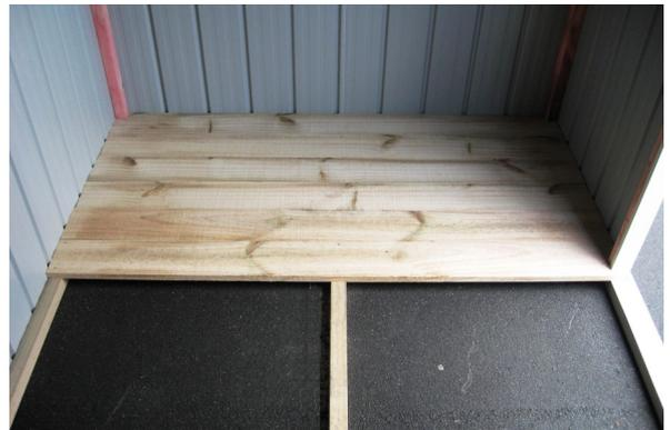
**Step 4:** Nail in each Floor Board, two 50mm nails in each end and two into Joist. Measure and cut Floor Flashing (110) to fit in between Door Jamb Flashings and nail in place using 50mm Clouts.
