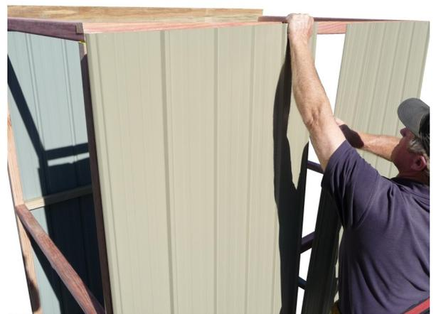
**Step 3: End Walls:** Position wall sheet with the LIP flush with the side of the stud and the top of the Wall Sheet is flush with the top of the Top Plate, tack in place. Tack in remaining 1/2 Wall Sheet. Repeat with the other end. If fitting a window, nail in Window Studs and Nog now. Refer to Window instructions.
