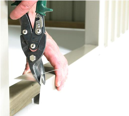
**Step3:** Measure and cut Doorstep Flashing (106) to fit in between Door Jambs. Position the Doorstep Flashing in between the Door Jambs at bottom of doorway, nail through top of flashing using three 30mm Clouts. Repeat with the Overdoor Flashing (105).
