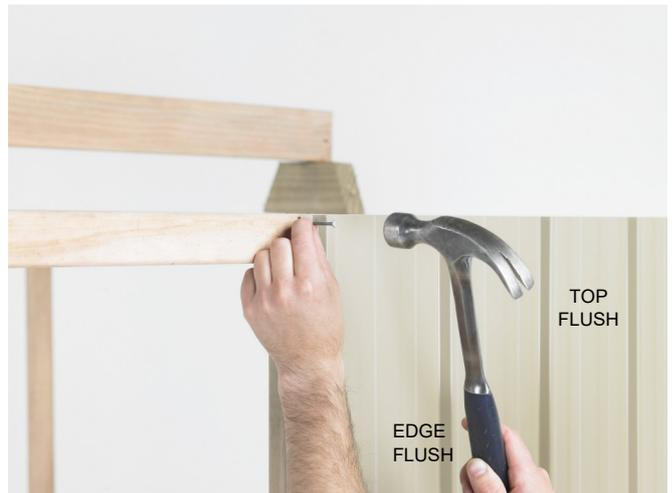
**Step 2: Back Wall:** Position the first Wall Sheet with the LIP on the right hand side. Ensuring the LIP is flush with the side of the corner Stud and the top of the Wall Sheet is flush with the top of the Top Plate, tack in place. Position the next Wall Sheet with the LIP on the right hand side. Overlap as shown in **fig 1**. Ensuring Wall Sheet is flush with top of Top Plate, tack in place.
