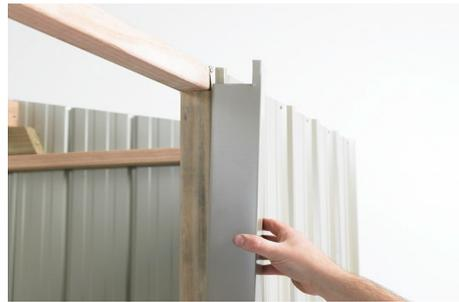
**Step 2:** On the left hand side of the front wall fit Corner Flashing (101) over Door Jamb Flashing and rib . With top of the Corner Flashing flush with the top of the Top Plate, rivet in place using six rivets.
