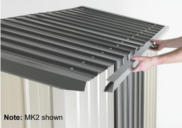
**Step 1:** Position Barge Flashing (A102) on gable ends. Position a Spouting (A103) and rivet to the Barge Flashing at each end. Repeat with other Spouting.
