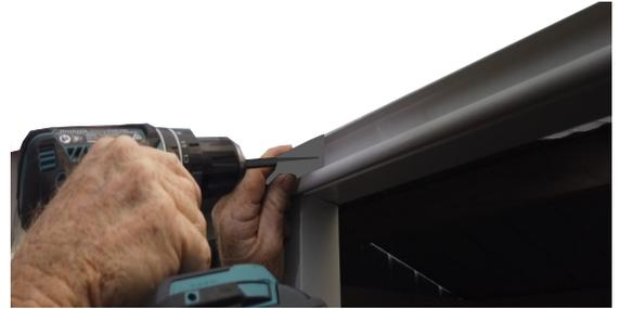
**Step 3:** Remove the Door. Pre-drill and screw another 2 screws between the centre screw and the rivets at each end (5 screws per track). Screw track using 45mm door track screws.
