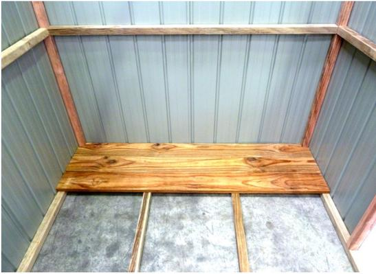
**Step 3:** Re-position Floor Board. Lay out remaining Floor Boards checking around Studs as you go. The last Floor Board may have to be cut to size.
