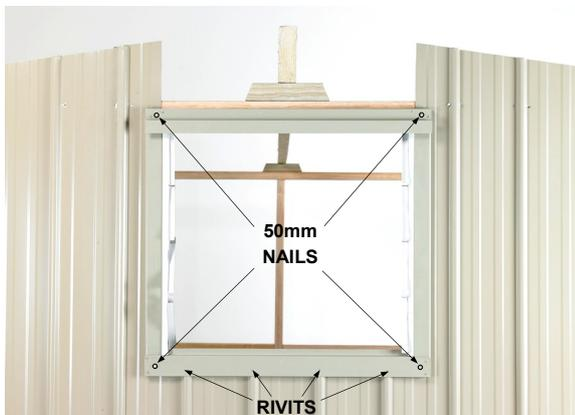
**Step 3:** Nail wall Sheets to window framing using 30mm clouts. (return to step 4 on page 7 and complete). Then fit Window Frame). Position Window Frame centrally on window opening and rivet it to ribs. Pre-drill holes in each corner and nail Window Frame to framing, using 50mm nails.
