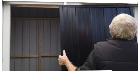
**Step 4:** Clean out ALL drill filings. Also make sure the Wheels are cleaned of drill filings. Re-hang Door.
