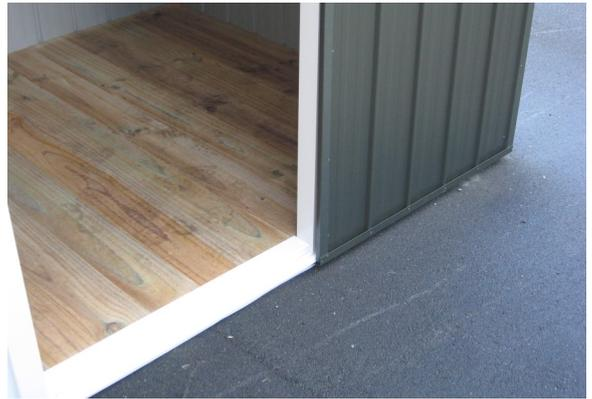
**Step 4:** Nail in each Floor Board, two 50mm nails in each end and two into Joists. Measure and cut Floor Flashing (110) to fit in between Door Jamb Flashings and nail in place using 50mm Clouts.
