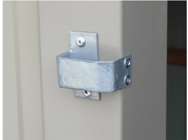
**Step 3** On the left hand Door Jamb, position latch so that the hook on the door handle will be secure and go in and out easily. Rivet in place with four rivets.
