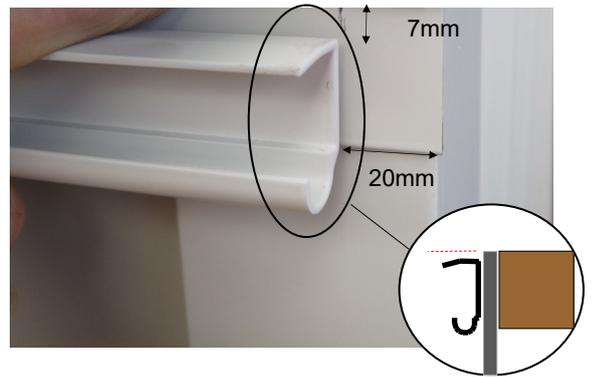
**Step 2:** Hang the door in the Door Track. At the right hand end of Door Track, adjust up or down so that the Door hangs parallel with shed. Fit one rivet at right hand end to hold in place. Repeat with left hand end of track.
