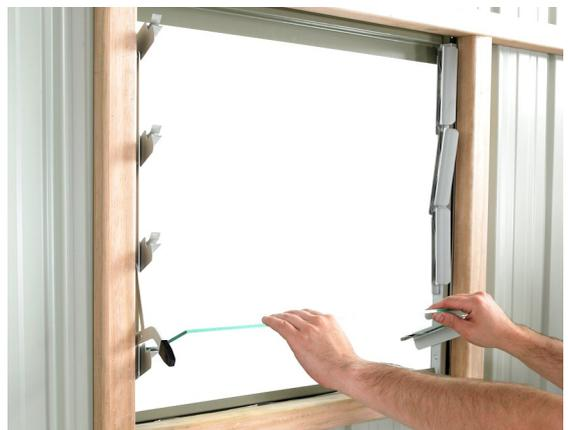
**Step 6:** From the inside of the shed, slide Louvre Glass into Louvre Units attached to the Window Frame. Bend up tabs to keep Glass in position.
