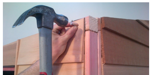
Note: Weatherboards will come to the edge at the corners. Unlike that shown above.
