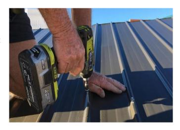
Step 18: Lay out remaining full roof sheets. Rivet these sheets together, 2 rivets per join, to make 1 large roof panel as shown in photo. Tack remaining front corner and back corner ensuring edge of sheet is flush with end of purlins and front overhang is correct.
