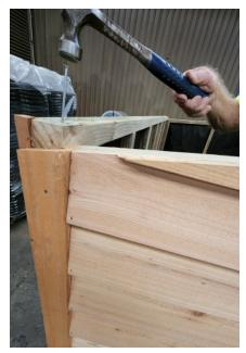
Step 11: Using 30mm clouts nail top cedar boards to Stiffeners (2-3 per board). Predrill holes to stop boards from splitting.
