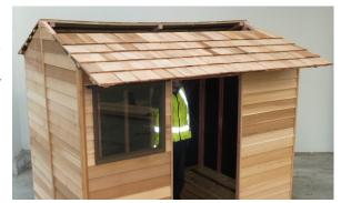
Step 15:Using 75mm tek screws, screw roof panels into end wall panels, (2 screws per panel), ensuring end of rafter lines up with centre of gable panel.
